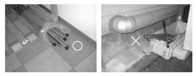
Store the pipes to be used indoors. (Warehouse at site or owner's warehouse) Storing them outdoors may cause dirt, waste, or water to infiltrate.
